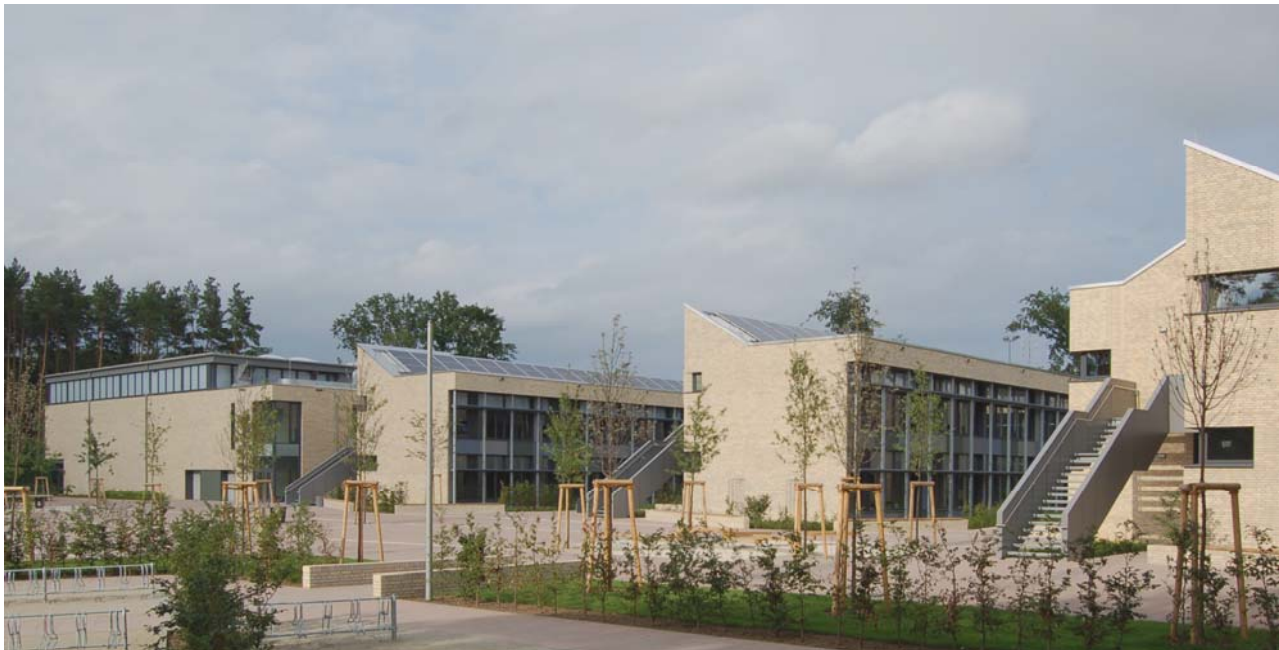
Figure 14: View from west
