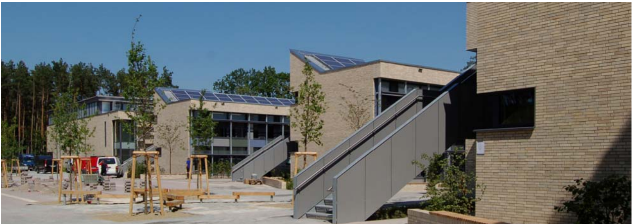
Fig. 1 Primary School Building, view from West
