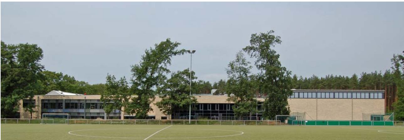
Fig. 11 View from east – facade of the specialist rooms, cafeteria and sports hall
